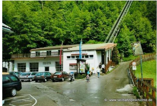
Figure 6. Valley Station of the Salzbergbahn Hallstatt before renovation (Sagen.at Forum, accessed May 2026)
