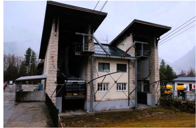
Figure 2. Cable Terminal, Valley Station, The Dachstein Krippenstein Seilbahn, April 2026 (Philip Nilsson)
