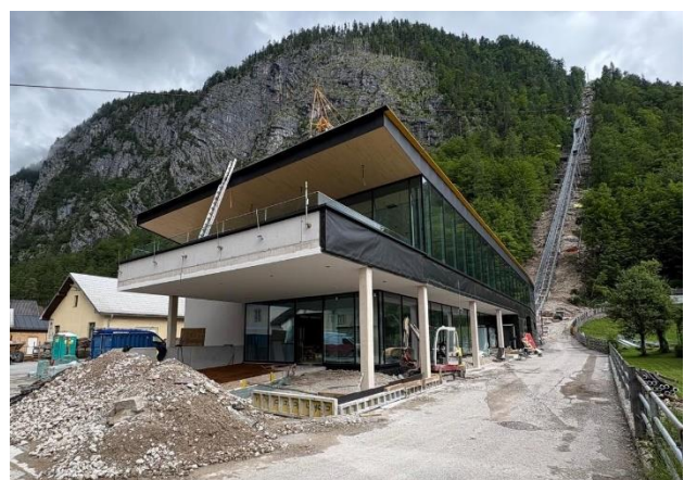
Figure 7. The new valley station of the Salzbergbahn Hallstatt nearing completion, June 2026 (Salzwelten.at, accessed June 2026)
